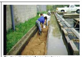
Routine cleaning of a perimeter or "Delaware" sand filter. This can be done from the surface, but deeper, vault-type filters will require confined-space entry procedures.
