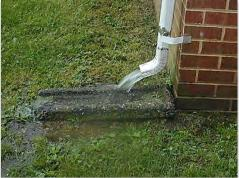
Both issues are fairly straightforward to address but involve communicating and working with property owners to explain the purpose of disconnection and how to properly maintain it. The second issue may involve some minor regrading or building low-profile berms to get water to flow to the intended disconnection area.
