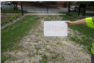
**Figure 12.3** Use a white board and digital camera to note SMP tracking #, date of inspection, and other forms of documentation. Alternatively, tag photographs using a smartphone
