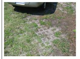
Pulling grass and weeds from the joints can damage parking surface if roots are firmly established in the bedding layer.
