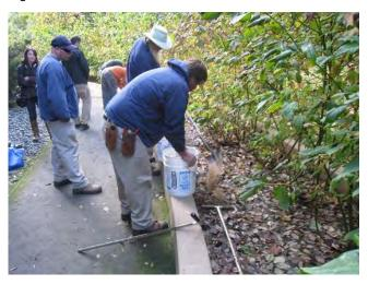
Adding sand to a wick drain. The vertical perforated PVC pipe has already been placed in the auger hole.
