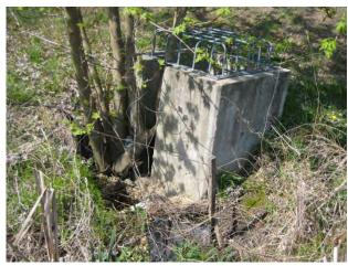
The pond outlet is clogged with sediment, trash, debris, vegetation, or is eroding, caving in, slumping, or falling apart.
