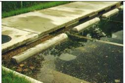
Standing water on the parking lot is evidence that this perimeter sand filter (under the sidewalk) is clogged.
