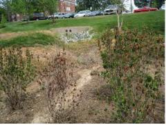
Water from the inlet at top of photo is channeling through the bioretention area.
