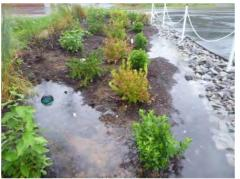
Water is preferentially ponding only at one end of the bioretention because the surface is not flat.
